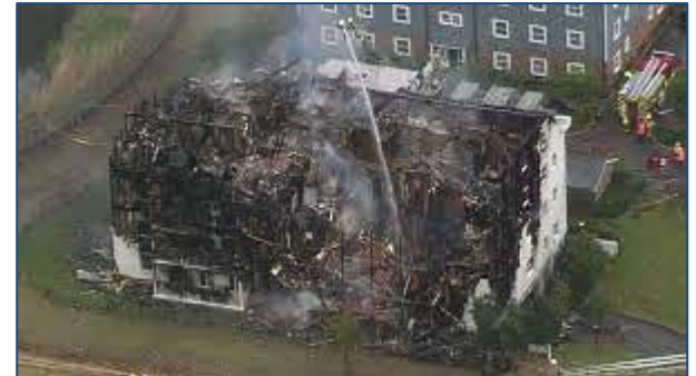
Richmond House September 2019
